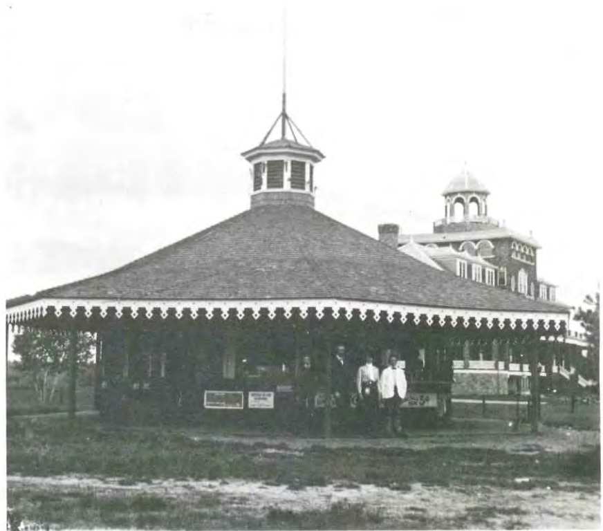
This is another view of the round house where snacks were sold and basket boys stocked up to sell refreshments all over the park grounds. The building replaced a tent that served the same purpose; neither are shown on the park map.
